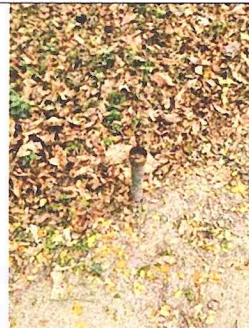
Photo: Earth-pit for DG-3's Body earthing.
