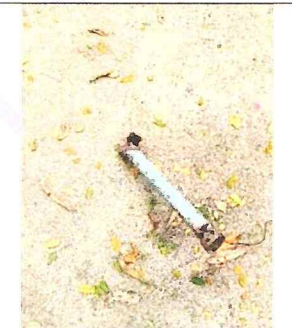
Photo: Earth-pit for DG-3's Neutral earthing.
